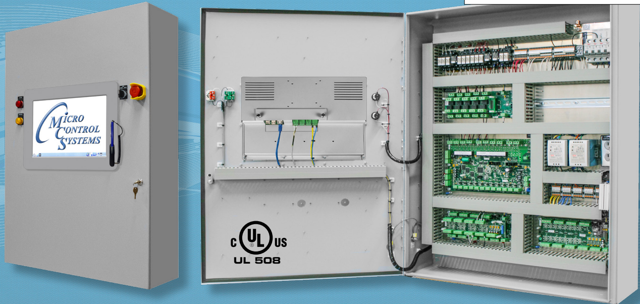
MCS-CENTRIFUGAL-12 Industrial Control Panel
